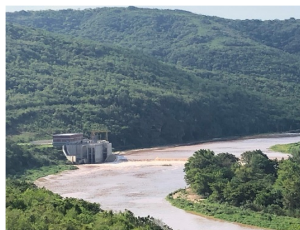
Photo showing the Umgeni abstraction works on Thukela River.
